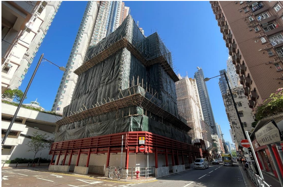
WOP's property project located at Nos. 120-130 Main Street, Ap Lei Chau
